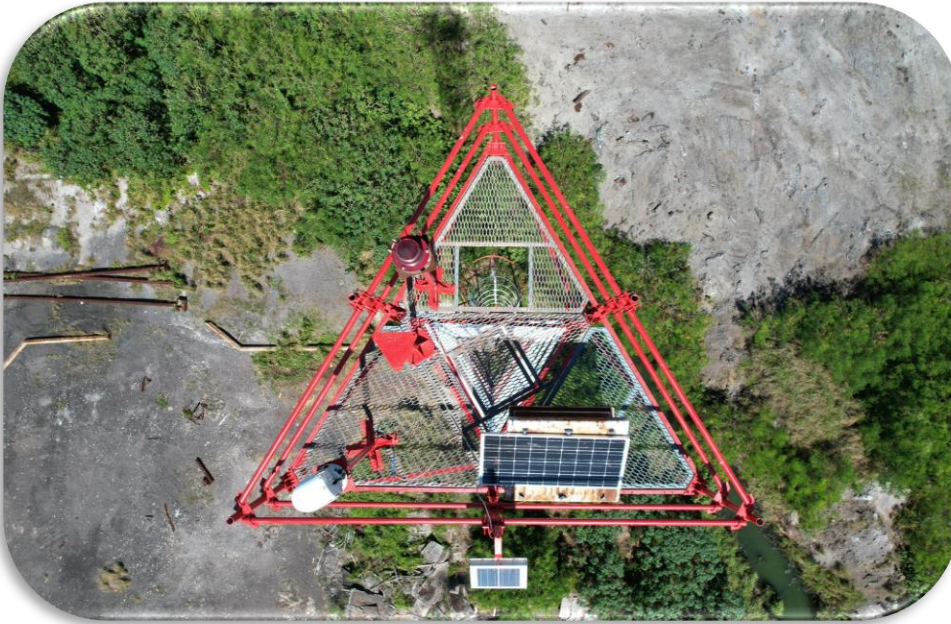
Aerial View Showing Solar PV System Installed by National Energy on the Rear Leading Light Tower
